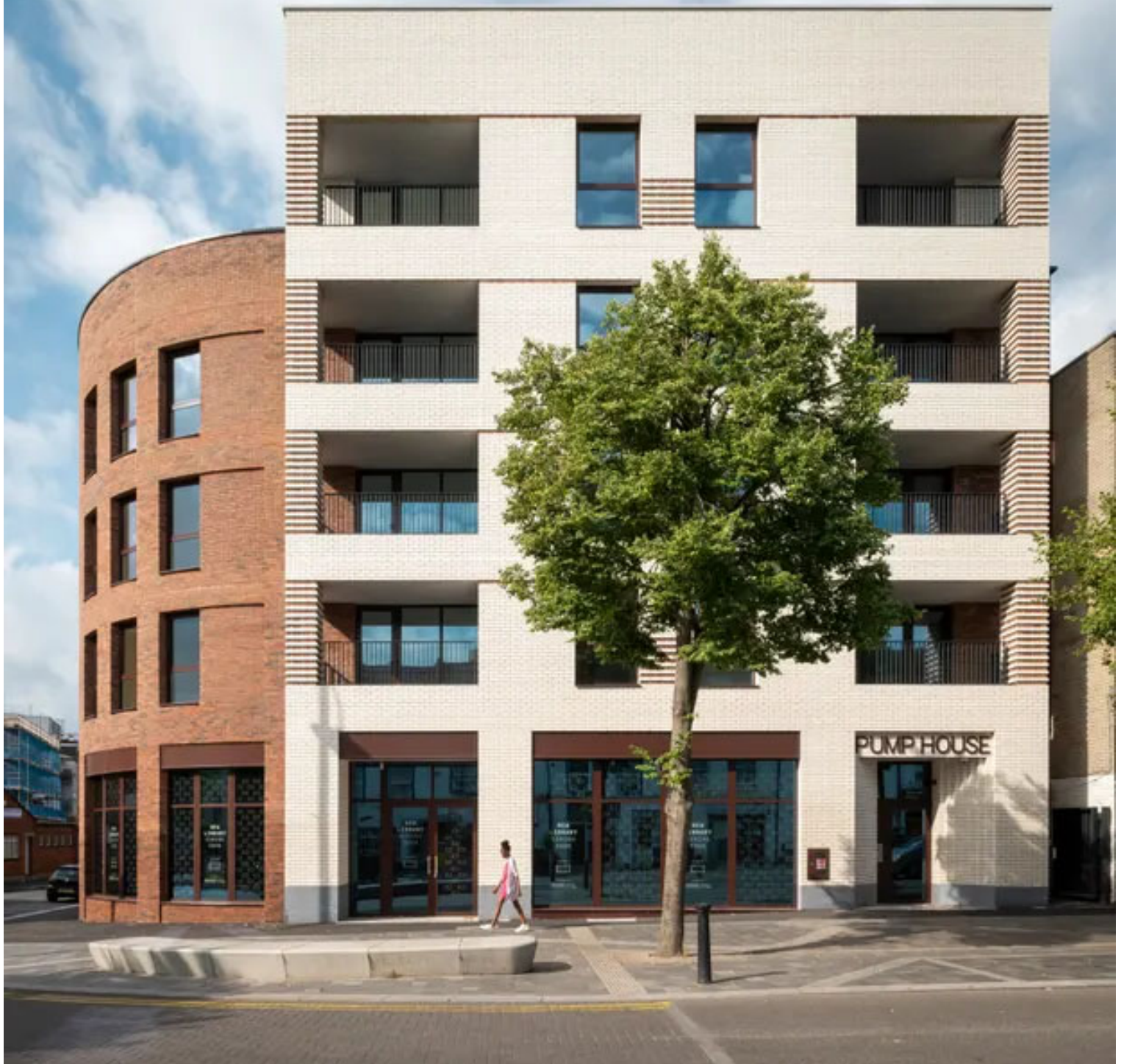
▲ Pump House by Common Ground Architecture and Brick by Brick. Photograph: Jim Stephenson
